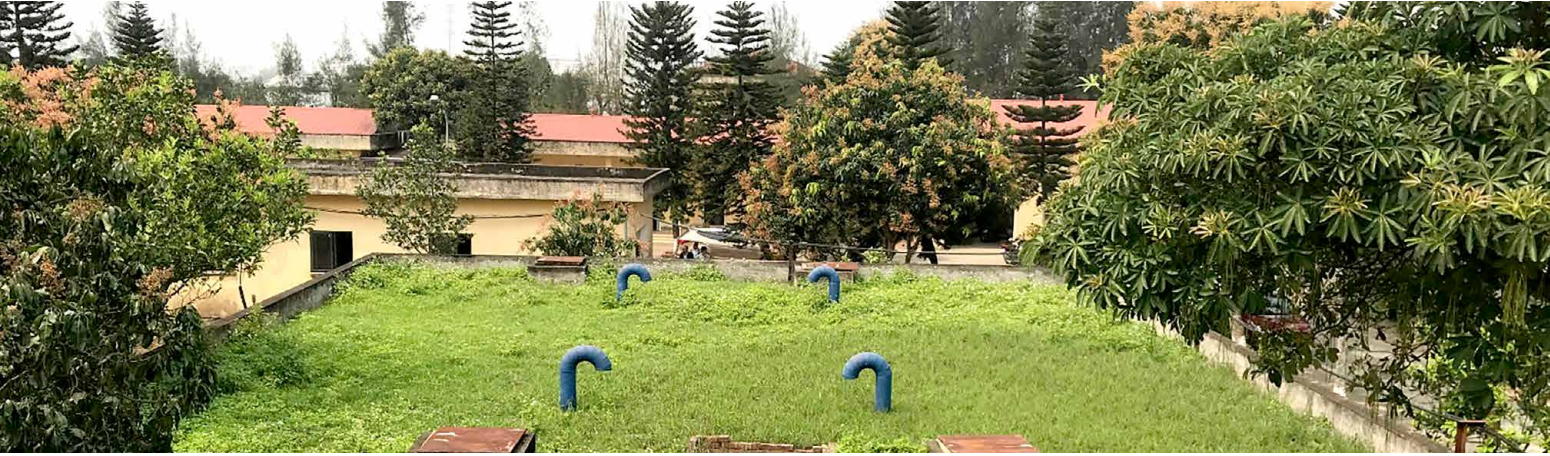
Clean water tank at the water plant Lien Bao commune, Nam Dinh province.
