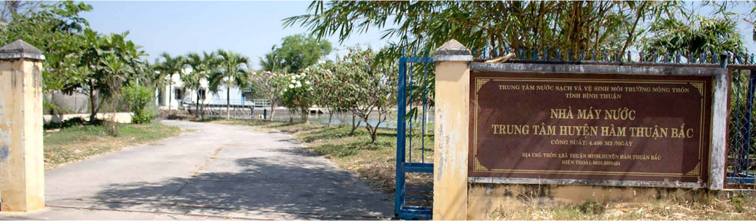
Central water plant of Ham Thuan Bac district, Binh Thuan province.
