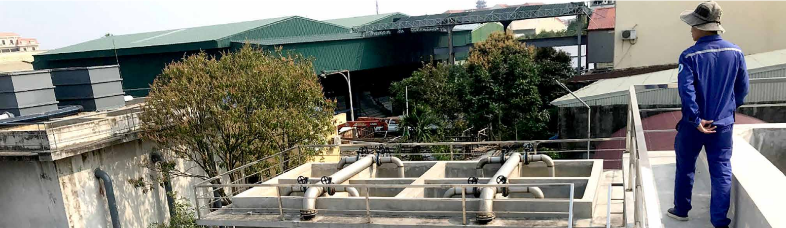
Water treatment area at Xuan Truong Water Plant, Nam Dinh province.
